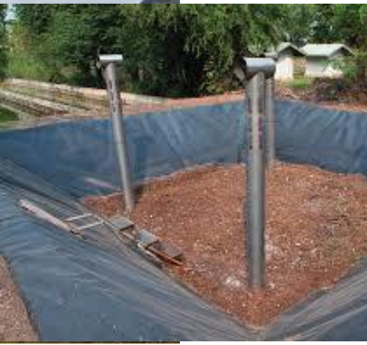
Unplanted sludge drying beds
